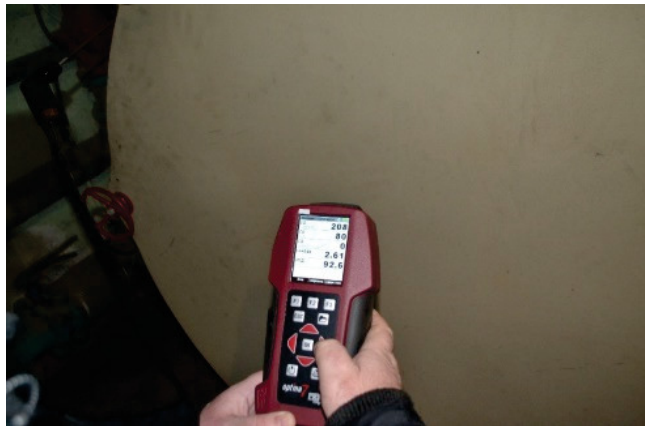
Figure 6. The results of measuring the efficiency a solid fuel boiler.
