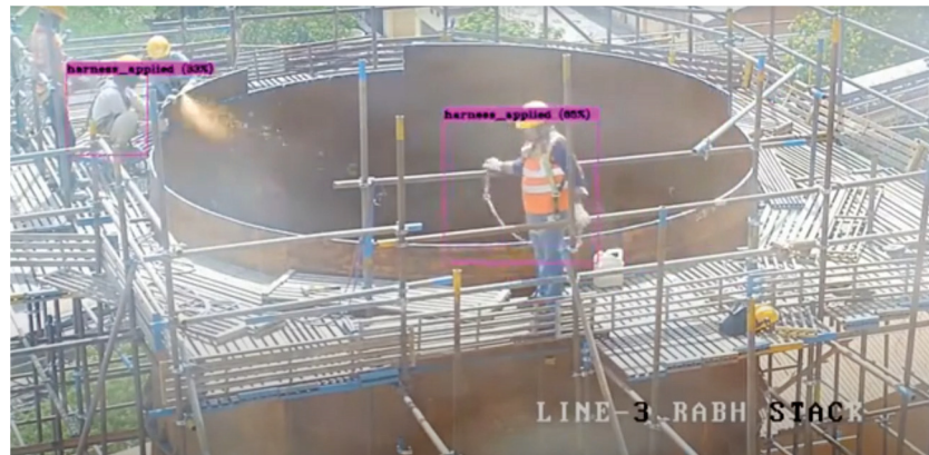
Figure 9. Work at Height [5]
